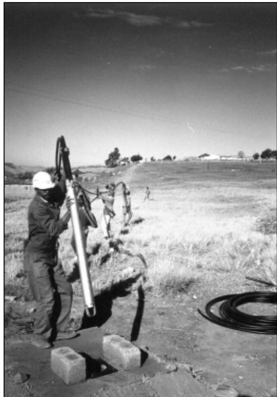
Community labourers install a Vergnet pump
