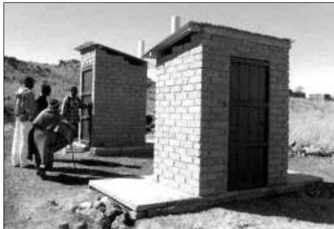
Community members examine two newly built VIPs
