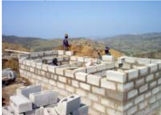
School toilet construction in the Eastern Cape
