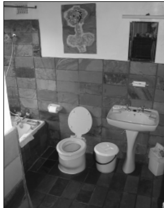
Urine Diversion in a suburban bathroom
